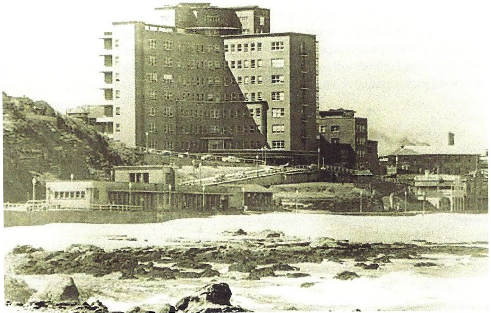
Royal Newcastle Hospital. The Nickson Wing overlooking Newcastle Beach was completed in 1950. (Photo courtesy Royal Newcastle Hospital Archive. © The RNH Heritage Committee.)
